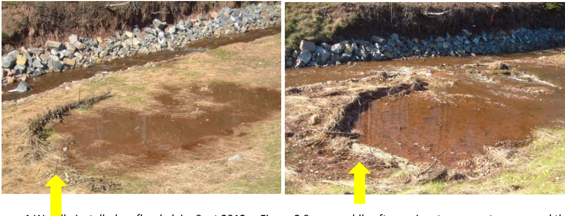
Figure 1 Wattle installed on flood plain. Sept 2012. Figure 2 Same wattle after major storm event rearranged the floodplain upstream. Wattle protected the lower portion of the floodplain and redirected the overflow back into the channel. October 2012.
