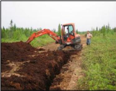
Figure 1a – Excavating a peripheral ditch
