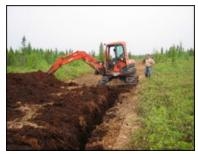
Figure 1a – Excavating a peripheral ditch
